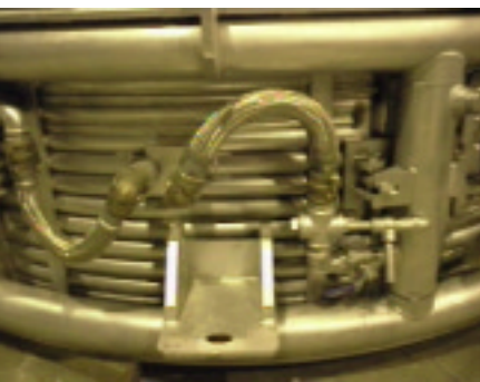
Water cooled ladle furnace roof
